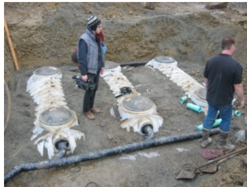
Rain tanks, prior to burial (tip of iceberg)
