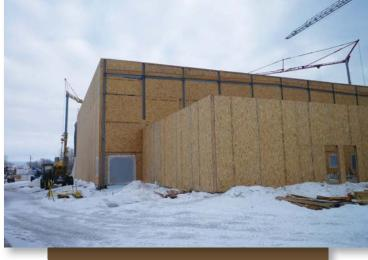
SIPs help create a tight, well-insulated building envelope for superior energy efficiency in any climate. Photo courtesy of BNIM Architects.
