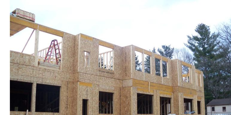
Six-inch-thick SIP walls helped DBA Architects reduce energy costs on the three-story, 48-unit building.
