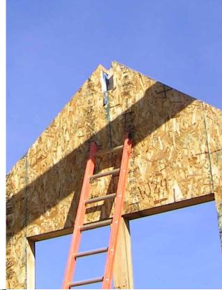
SIPs arrive at the jobsite with window openings and other features prefabricated. (Above) Wall panels are notched to accept a glulam ridge beam that supports the roof.
