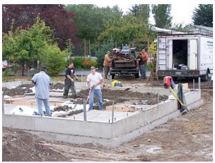
On Day 9, the lean mix has firmed up enough overnight for the plumber and electrician to show up and dig utility ditches which go in under the slab. Placement is critical; the main conduit that goes up into a 2 x 4 hallway floor has to be with in an inch of plans. Once the pipes and conduits are in place, the lean mix will be shoveled in again and smoothed over to give a good base for the foam under-slab insulation and the slab.
