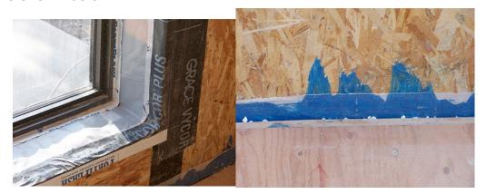
We were confident that the windows were not going to leak. The Vycor did not stick to the concrete slab, so we had to come up with something else to seal the perimeter at the floor. We used the mastic that Premier supplied to glue the sips panels together and put it between the OSB wall and the vapor barrier under the plywood subflooring as shown in the picture above. This caulk will remain flexible and the drywall will provide additional insurance.
