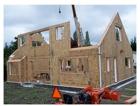
The top image shows the east wall being lifted in place and the bottom image shows the house with all the walls up. The whole process took 3 1/2 days with 3 workers. Keep in mind that the insulation for the walls is also complete and there is a complete nailing surface on the inside of the exterior walls.
