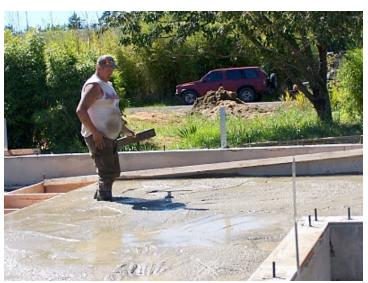
In the 5th image, the footings and stem wall is complete. Because all the earth was scraped off to the depth of the bottom of the footings, we need to backfill. The backfill needs to drain well, and provide a good base for the vapor barrier and foam, which come next. We elected to go with a lean mix of sand and cement, and needed 4 truckloads of 9 cubic yards each on Day 8! The wood forms block out an area below the ridge line in which we need to have a thicker slab.
