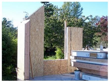
On day 26, the 10" wall panels arrived. They consist of inside and outside layers of 7/16" OSB and 9+ inches of high density EPS which has an insulation value of R-5 per inch. I held my breath during the unloading because of the bow in the 2  $\times$  4s supporting the load (2nd picture). Three hours after delivery, the SW corner is up.
