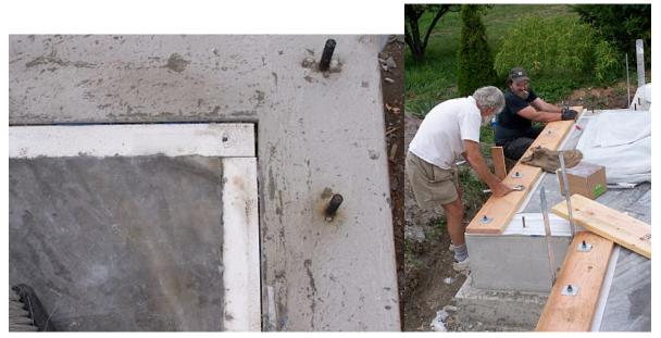
The top image shows the foam insulation between the slab and stem wall. The bottom image shows Charles and Mike installing the sill plate over a thin foam layer (<u>Sillseal</u>). Keeping air leaks to a minimum is a critical step in passive house construction. To make up for any roughness on the top of the stem wall, there is a bead of mastic between the concrete and the Sillseal.
