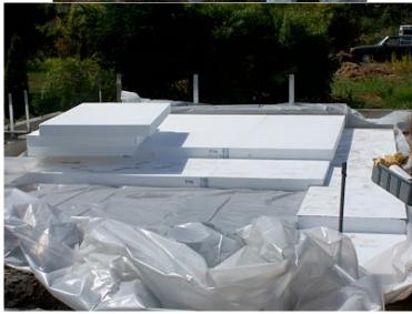
You're looking at \$3k of expanded polystyrene foam which will give R40 under the slab. This is 5 times what code requires and is the first significant additional expense of a passive house over a conventional house. My builder Charles in the yellow slicker can't wait and is getting ready to put in the foam in the SW corner of the house where there are no utility ditches on Day 9. The vapor barrier goes under the foam and will go under the sill plate.
