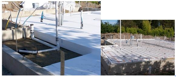
The first image shows the 10" of foam under the slab and the second image shows the rebar in place. There is a vapor barrier between the foam and rebar. The shaded area in the second image is where the slab will be thicker to support the weight under the ridge beam. Here we have no way to avoid having the foam under this portion of the footing. We're ready for the concrete!
