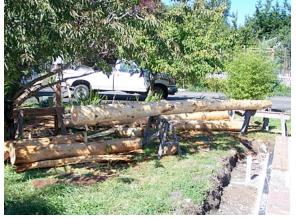
Before the roof panels go in place, we need a ridge beam, which is supported on two 21' high fir logs. The top picture shows us hauling the logs onto a trailer using a come-along. We got five, of which 2 will support the roof over the front porch. That was a good morning's work. I peeled them at the site as shown in the second picture, and two posts were hoisted in place using the crane. In the lowest image, the ridge pole is placed on the log posts.
