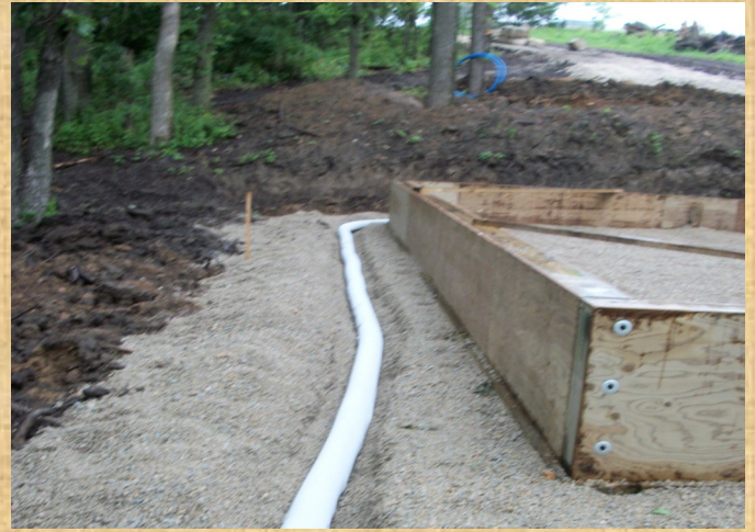
Frost Protected Shallow Foundation with 2' x 6" SIPs
