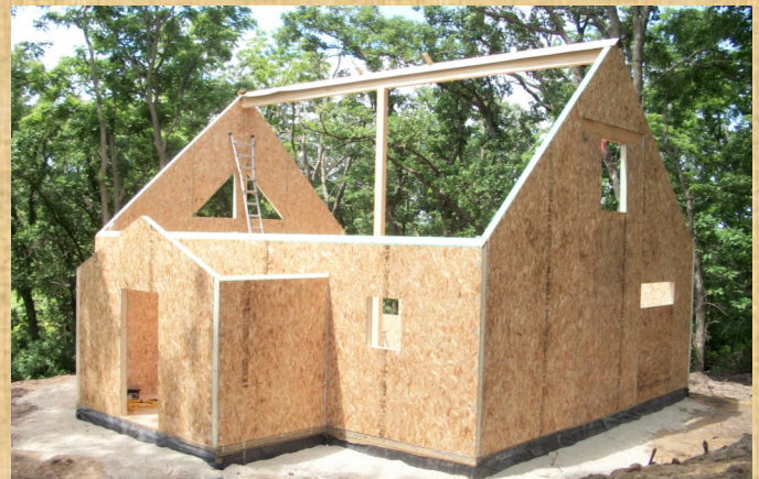
Ridge beam in place
