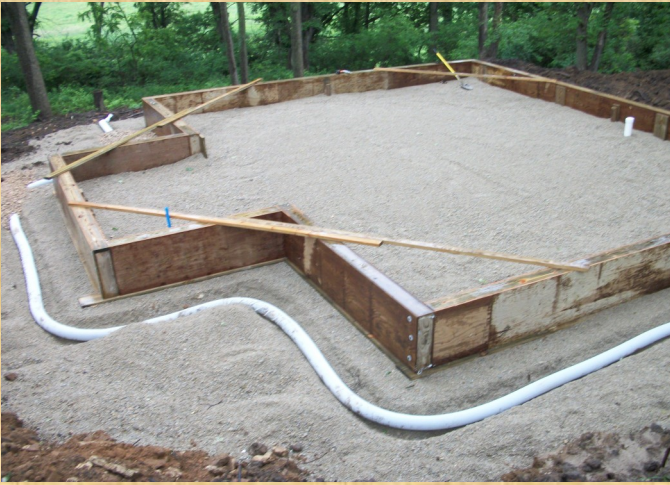
Frost Protected Shallow Foundation with 2' x 6" SIPs
