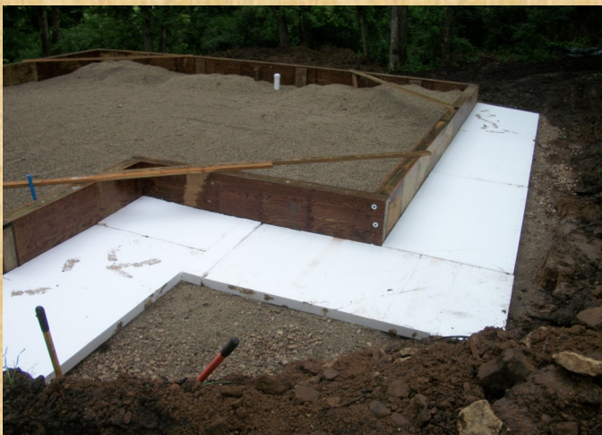
4" Horizontal Insulation
