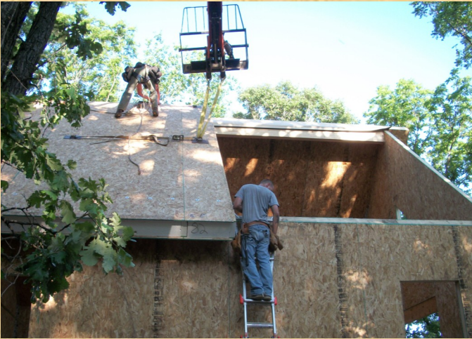
Setting SIP Roof Panels
