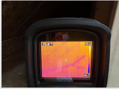
SIPs roof in bedrooms and behind kneewalls appear well sealed
